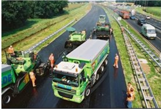
Figure 4 Test section two layer porous asphalt
