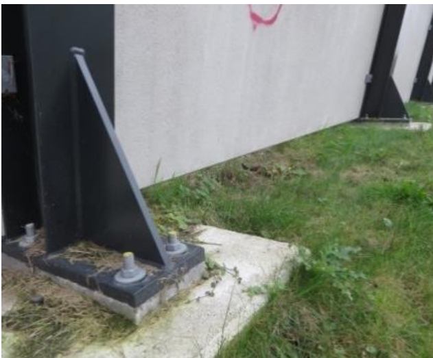
Figure 2. Example of drainage gap under noise barrier (A2 Nieuwegein)
