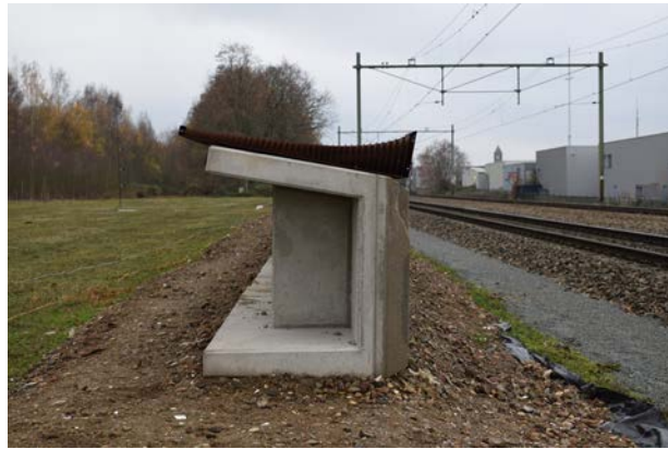
Fig. 1. Diffractor on top of a low noise barrier.
