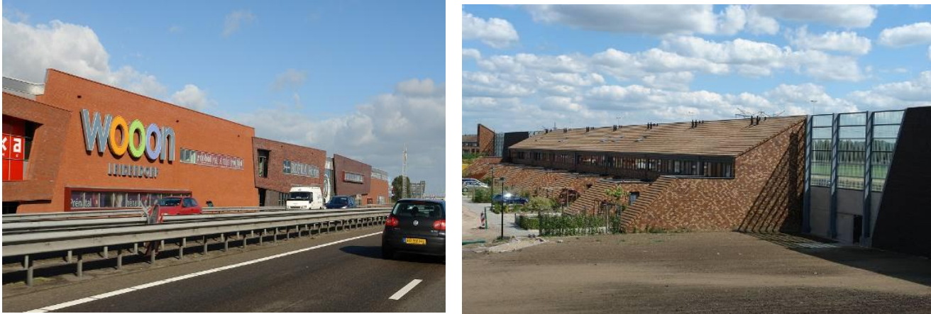
figure 21 Examples of barriers that are combined with other functionalities. Left: shopping areas, right: housing areas.
