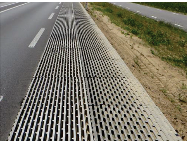
Figure 2. Whisstone diffracting elements variant 2 (section 2)
