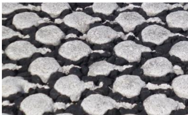
figure 6 Example of a dot marking on SMA with different dot heights
